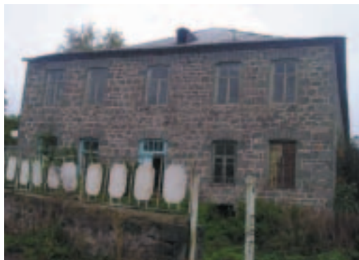
Exterior of the Tsintskaro, Georgia health post.
